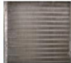
Coil after UV light application
