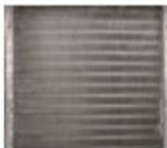
Coil after UV light application
