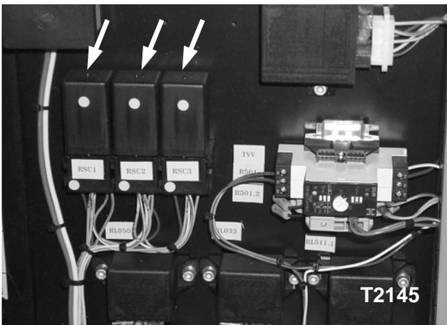
**Figure 2 – T2145 brake pad wear indicator relays (from left to right):**
