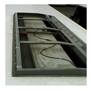
Step 2: Pry up on end of cover being careful, because cover is stuck down to the cross beams with silicone.
