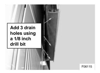
Figure 27: Sliding lift door drain holes
