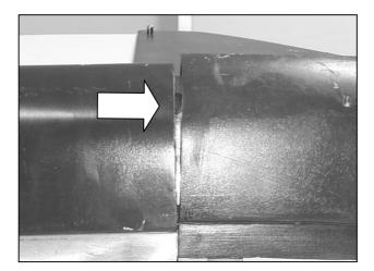
Figure 2: Mock-up showing cap and roof edges not flush and true
