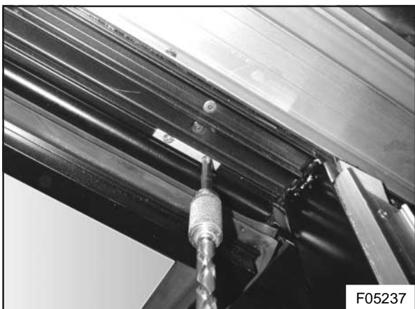
Figure 8 : Removing an end-stop
