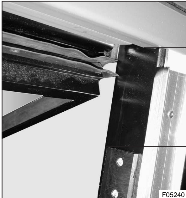
Figure 12 : Installed window guide
