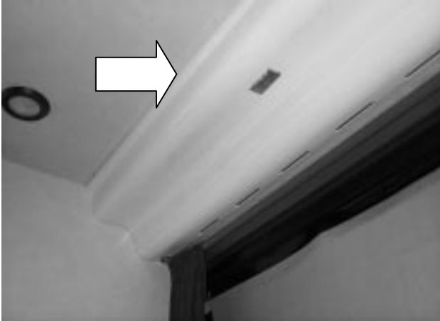
Figure 14: Push the outlet molding towards the window to remove it from the retaining strip.
