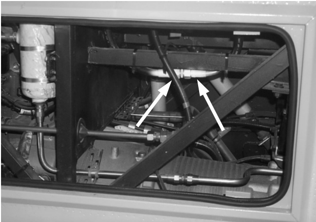
Figure 7: T2145 - Behind the RH engine compartment side door - engine compartment to central tunnel line connection. Check two crimp fittings.
